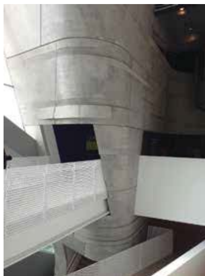
Precast panels were digitally modeled in the design assist process which allowed greater integration/coordination with other building materials. All photos: Gate Precast.
