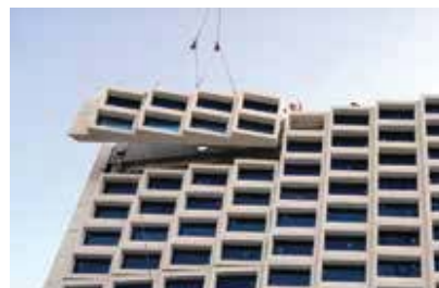
Topping out enclosure with last window panel. Photo: DPR Construction.
