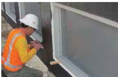
Prior to delivery, each precast panel was pre-glazed, caulked, inspected, and applied with waterproof coating on the back face.
