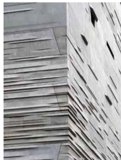
Precast panels were digitally modeled in the design assist process which allowed greater integration/coordination with other building materials. All photos: Gate Precast.
