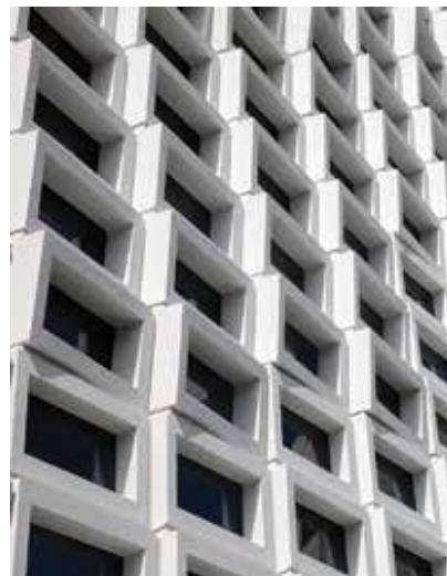
Actual photo of precast window openings that tilt in multiple directions.
